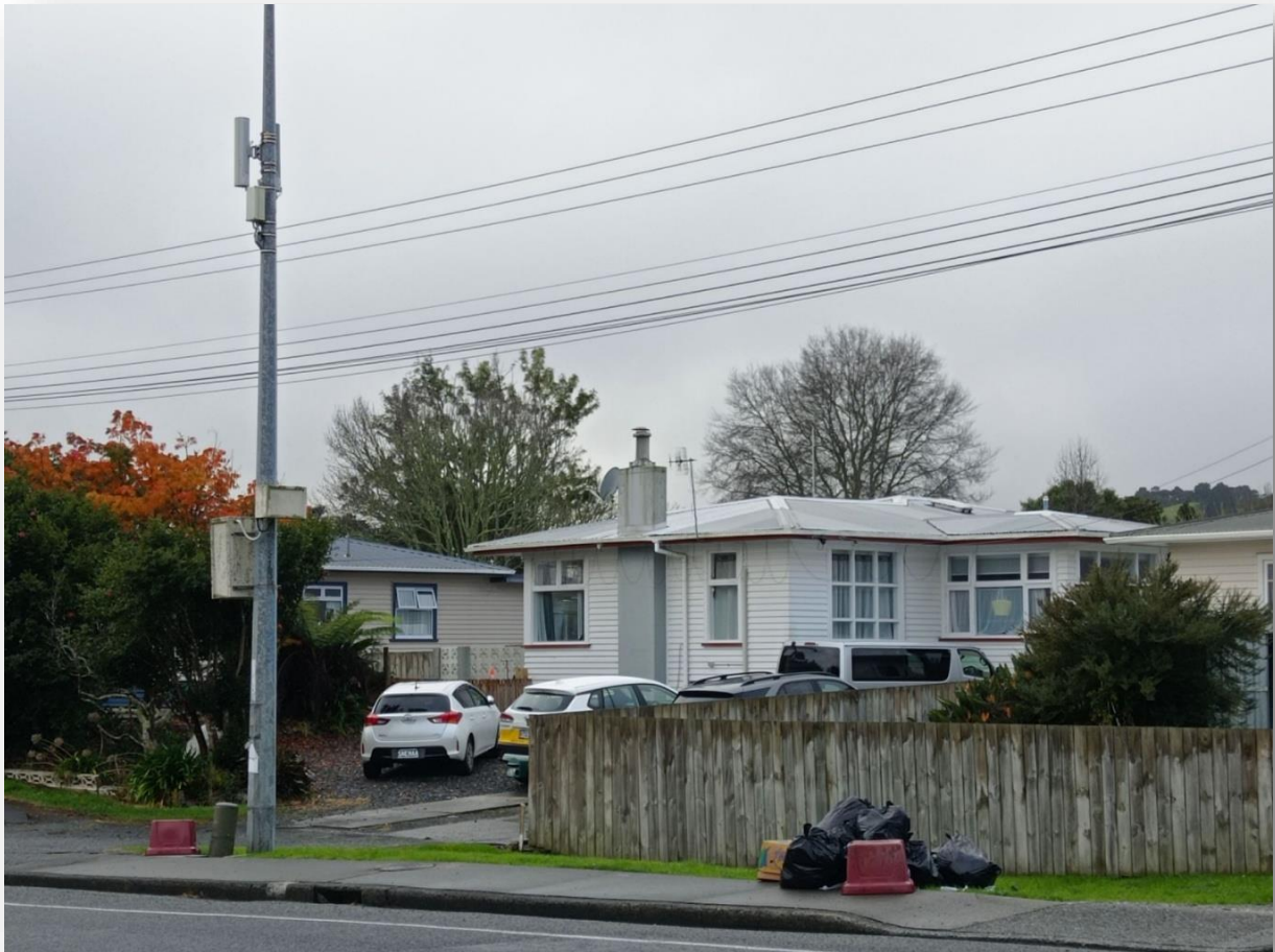
Onerahi (Whangārei) 5G mini cell tower directly outside residential home – photo taken by the author
