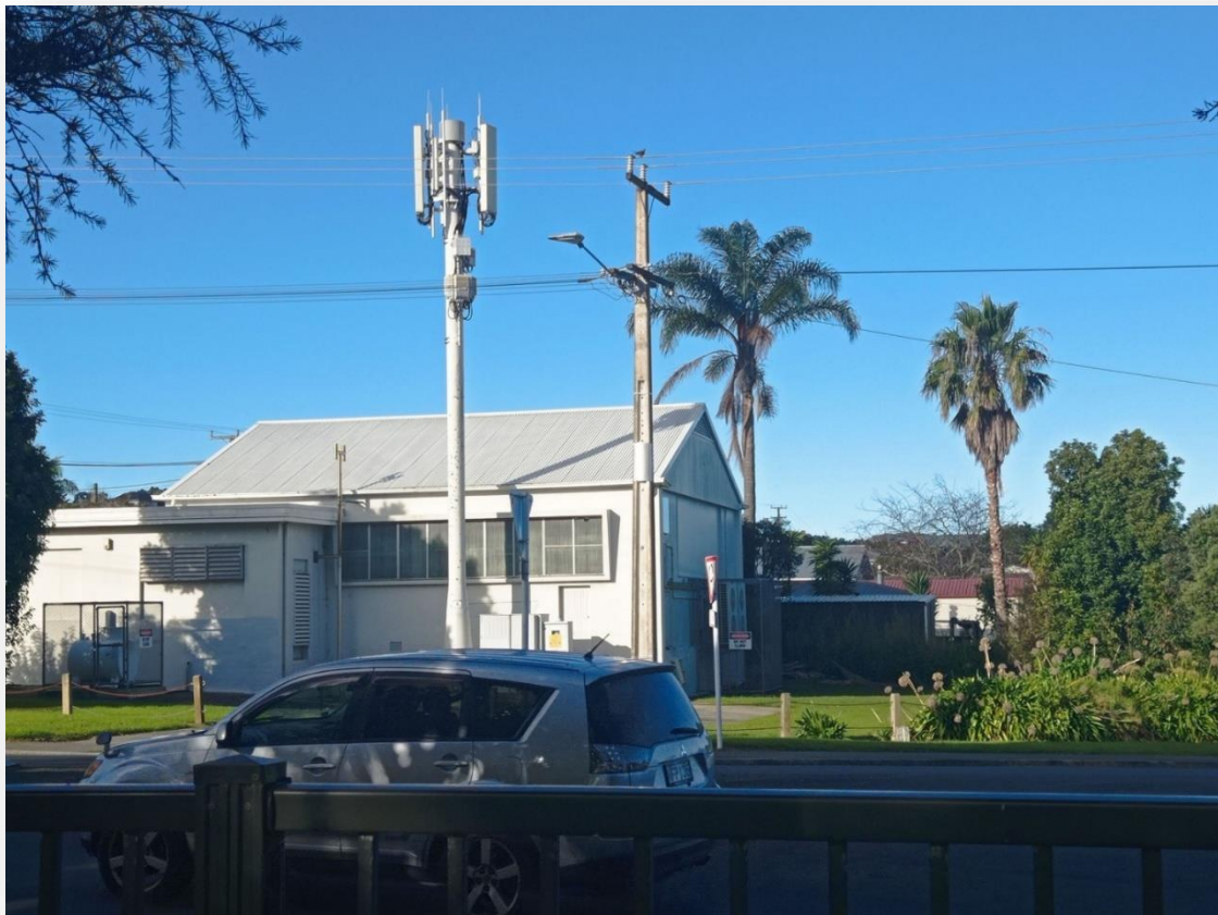
4G-5G mobile (macro-cell) cell tower only about 50 metres from the boundary fence of Onerahi Primary (Whangārei) – photo by author
